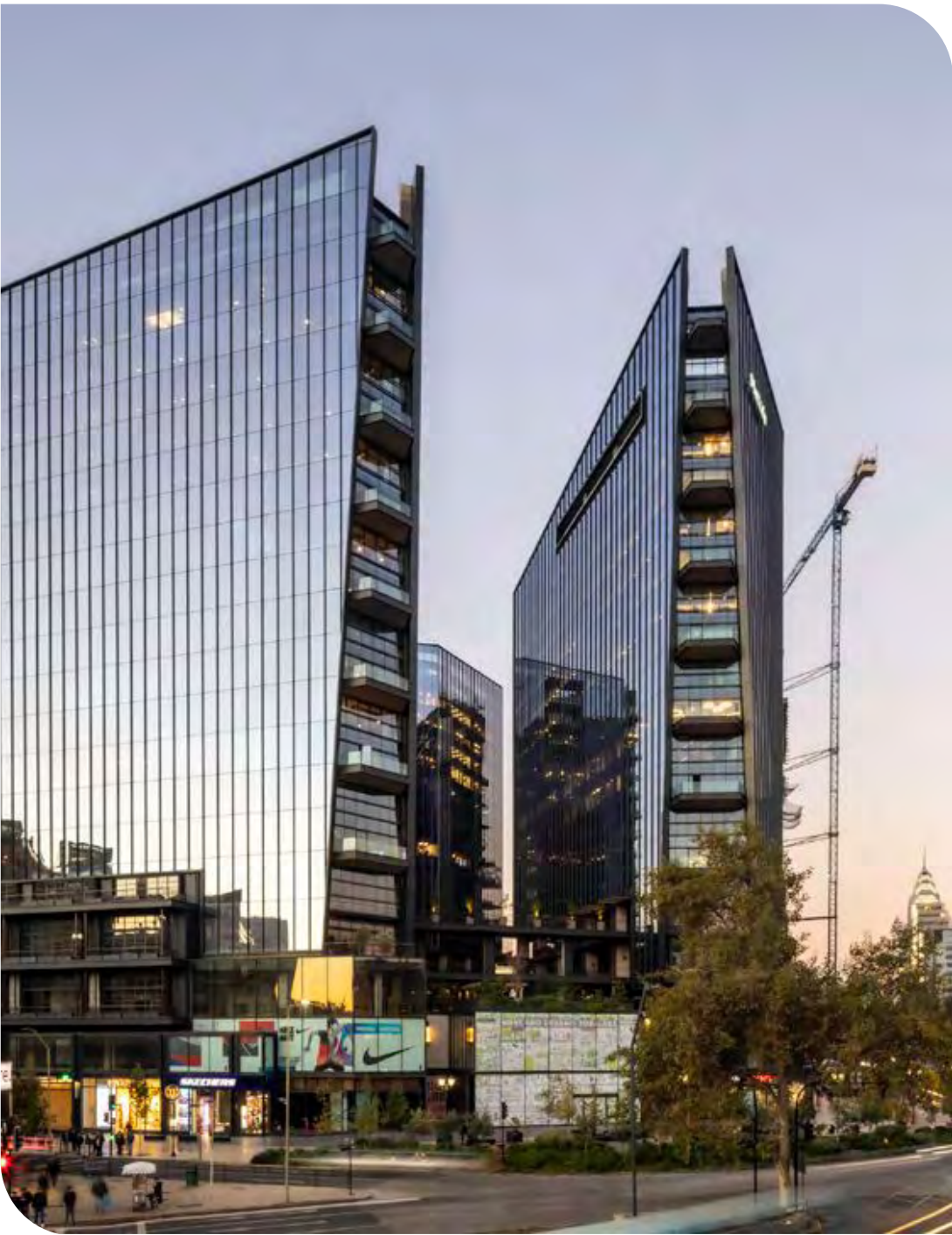
View of MUT building / Encomenderos street access.
